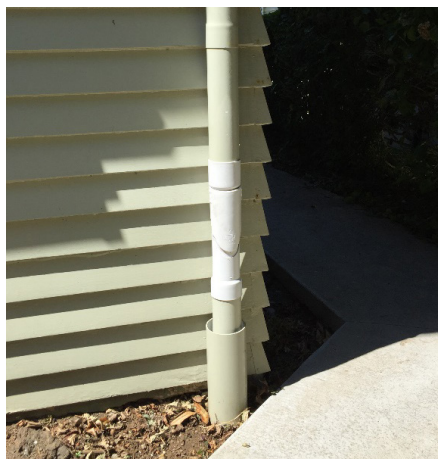
A proprietary diverter in the closed position.
