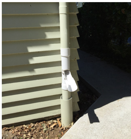
A proprietary diverter in the open position.
