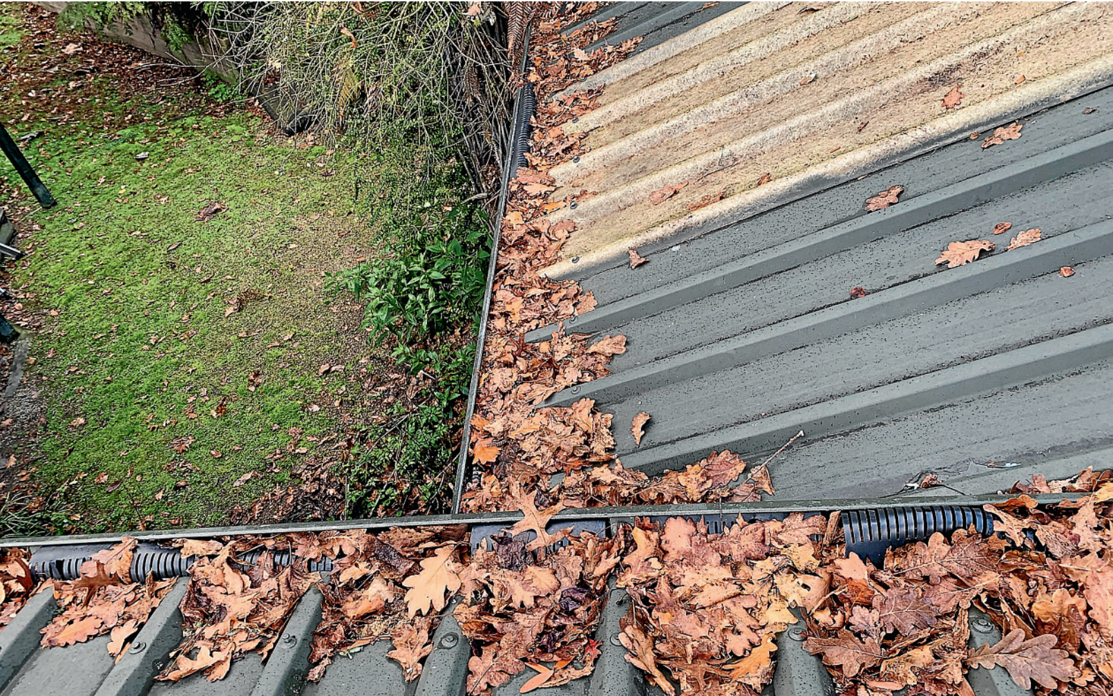
A leaf blocking device that sits in your guttering will allow the water to flow while ensuring any debris like leaves can't sit and block the gutter. PHOTO: FOURSEASONS GUTTER PRO.
